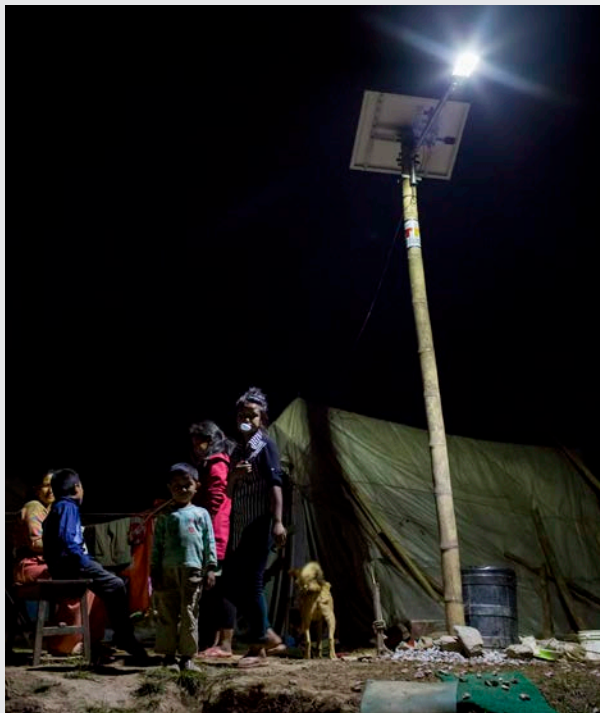
Solar street light in a refugee camp, Nepal
